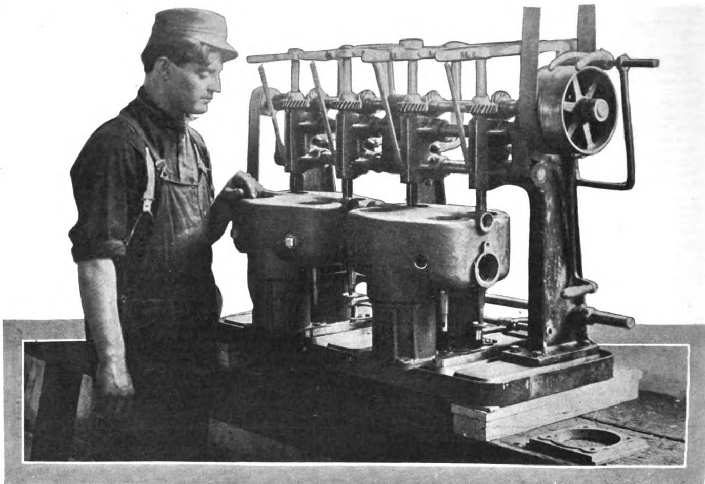
Machine used for the grinding of valves in the factory of the National Motor Vehicle Company at Indianapolis, Ind. It will do the work on a four-cylinder motor in 30 minutes
